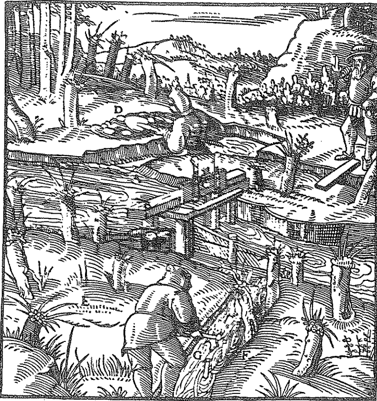
A—RIVER. B—WEIR. C—GATE. D—AREA. E—MEADOW. F—FENCE. G—DITCH.
